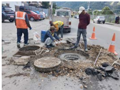
Raising and lowering of manholes in various locations
