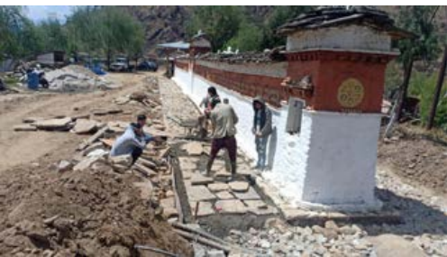
Paving of footpath
