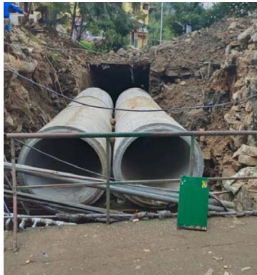
Installation of hume pipes
