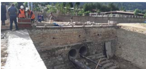
Installation of hume pipes and reconstruction of road
