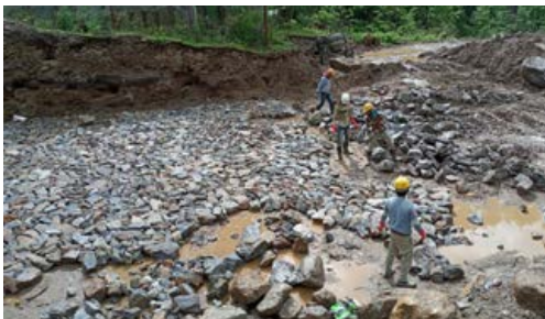
Laying the foundation for 3.5 MLD WTP in Chamgang
